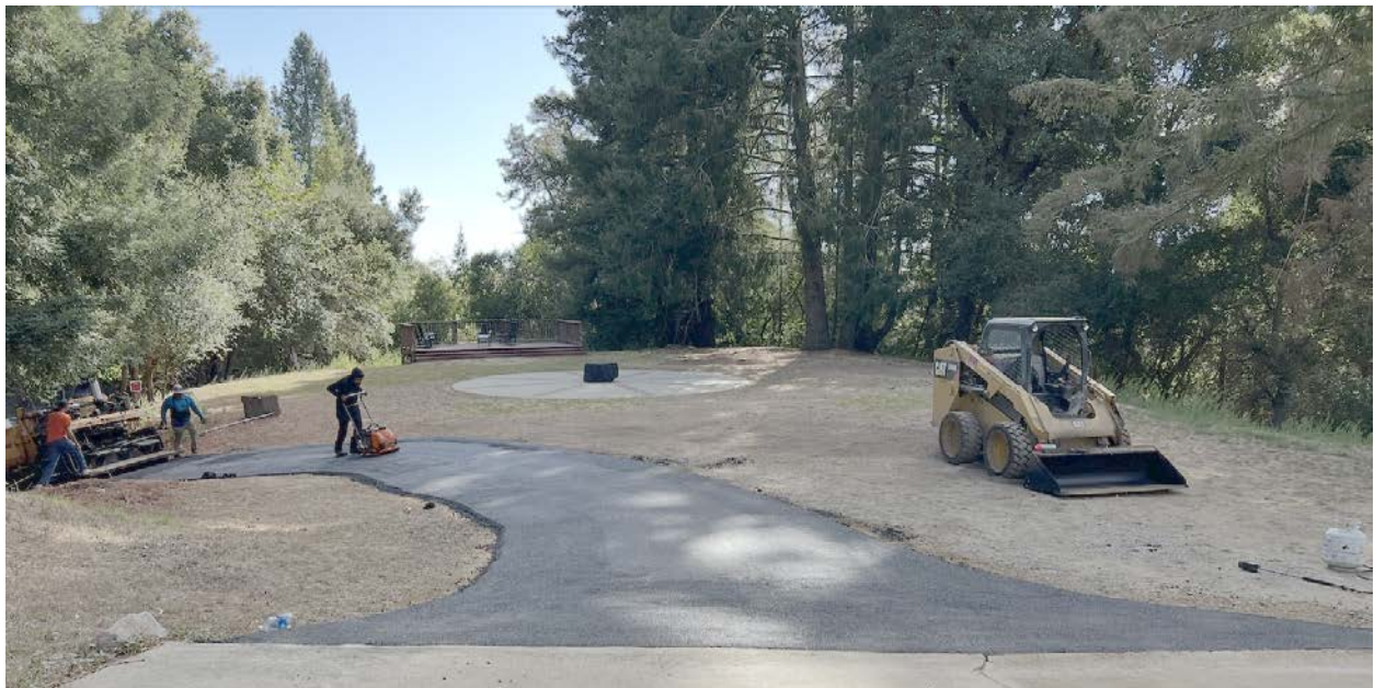
Paving the Eastern Cabin Road
